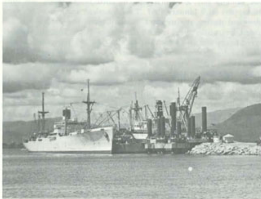
A DELONG PIER under construction at the Cam Ranh port facility.
