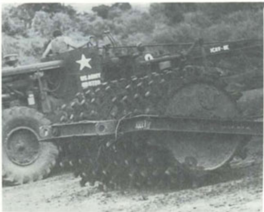
SHEEPSFOOT ROLLER compacting a runway extension at Bu Dop airstrip.
