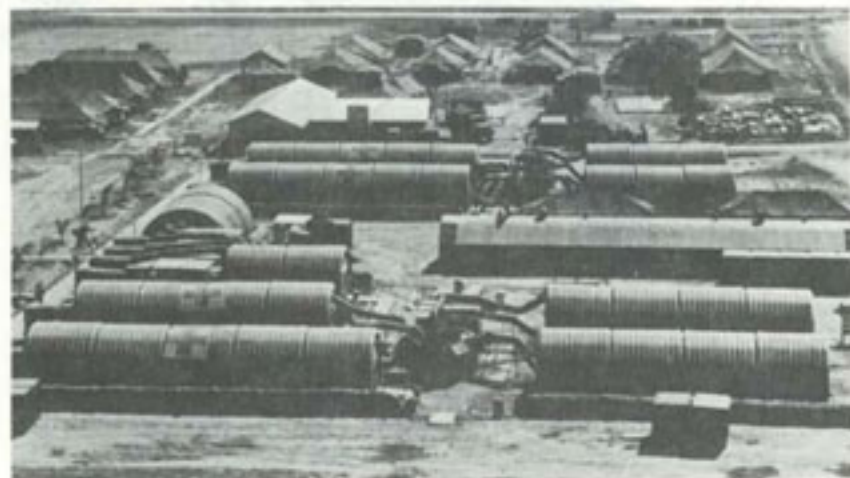
SPIDERLIKE DUCTS provide air to MUST hospital complex from centralized air-conditioning units.
