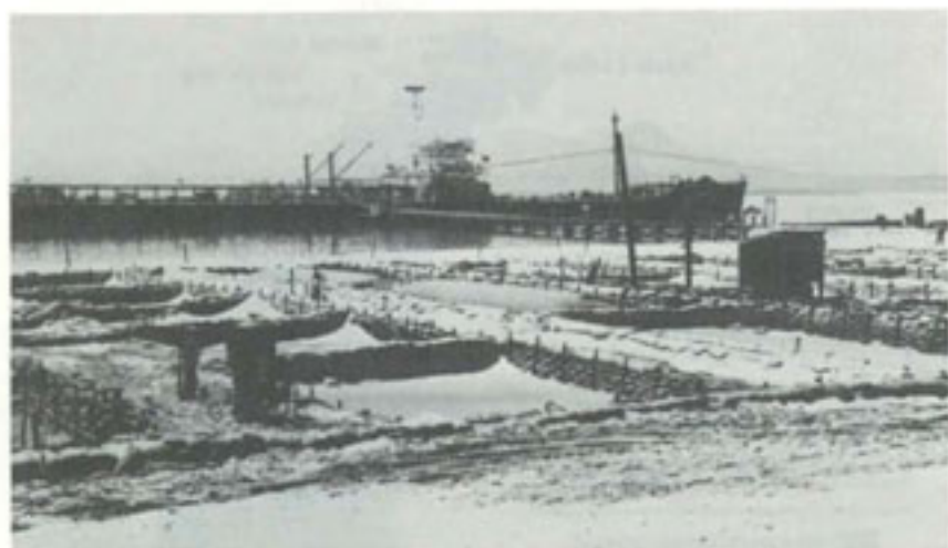
BLADDER FUEL CELLS lie in sandbag revetments at the Cam Ranh POL facility.
