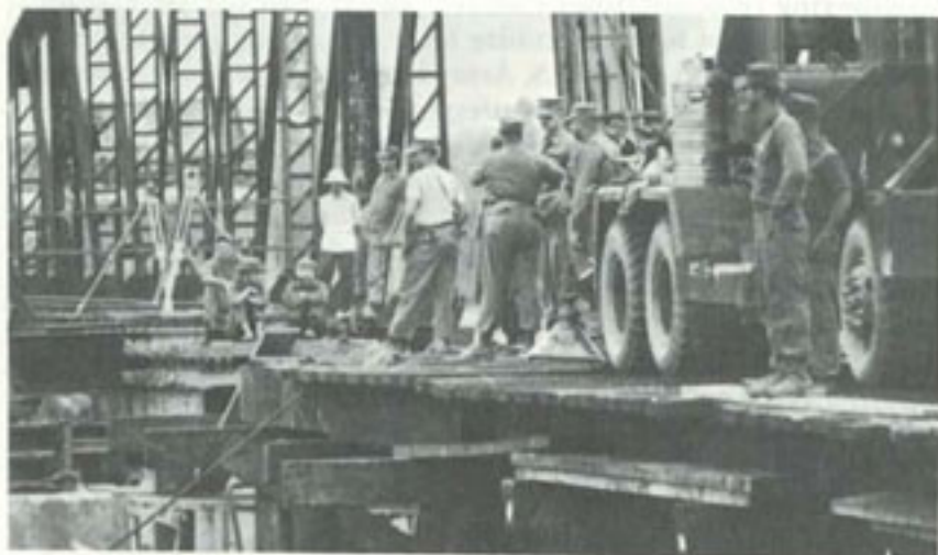
SEABEES responsible for bridge construction in I Corps.
