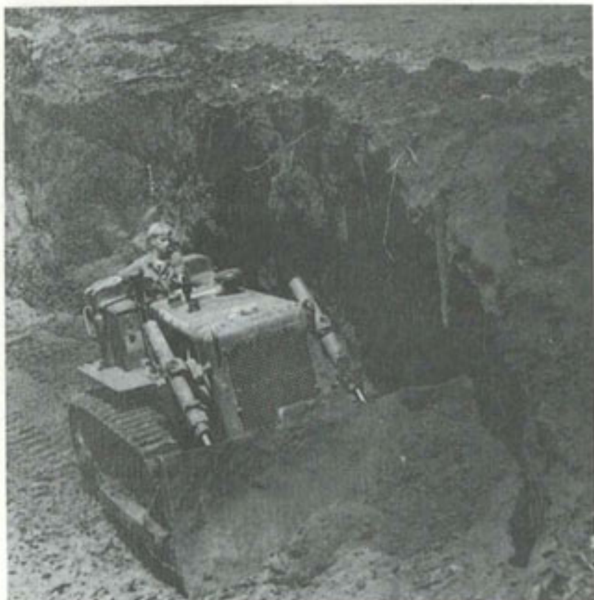
D-7 TRACTOR working a borrow pit.
