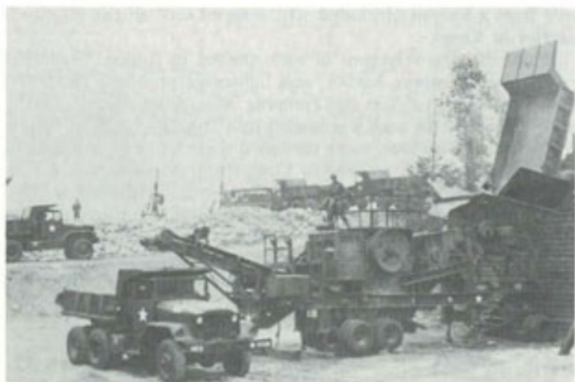
ROCK-CRUSHING OPERATION, essential to virtually all phases of construction.
