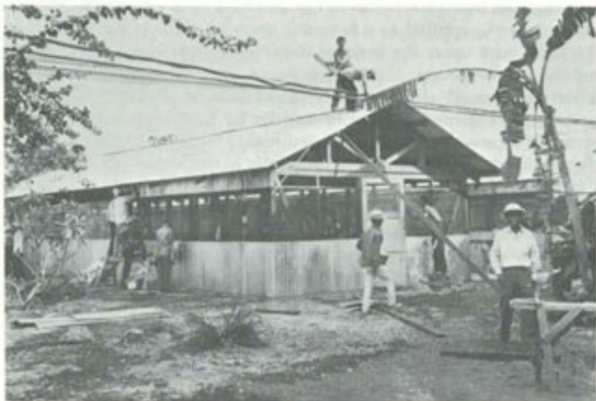
VIETNAMESE CONSTRUCTION WORKERS erect a tropicalized hut at Tan Son Nhut.
