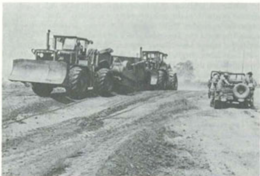
SCRAPERS PREPARE A RIGHT OF WAY before crushed rock is dumped.
