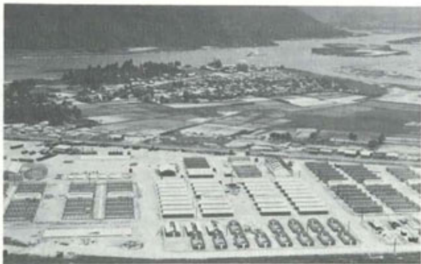
A COMPLETE SELECTION of wood, aluminum, and steel buildings under construction.
