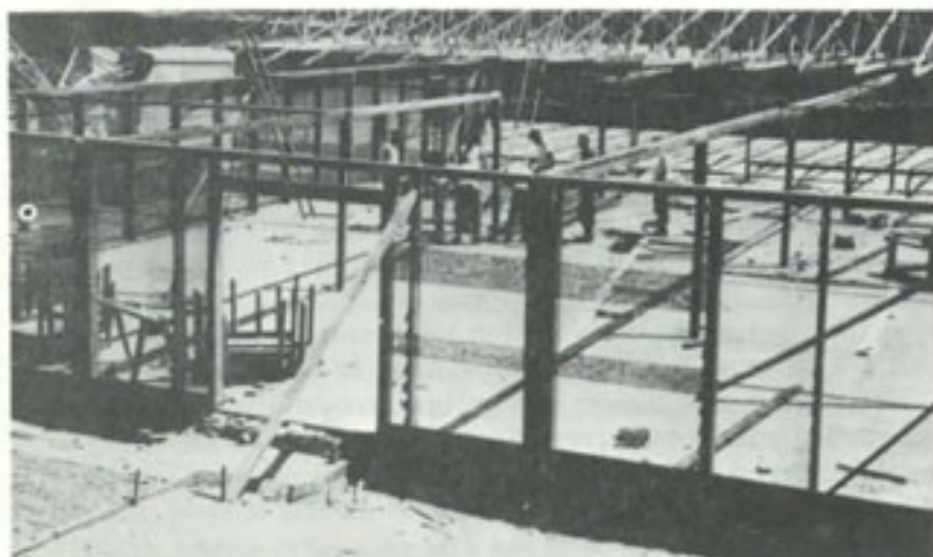
QUARTERS rise on concrete slabs at Long Binh.
